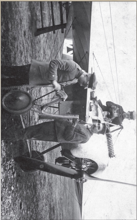
Ernest Udelt inspects a box of 7.7mm ammunition as it is loaded into the external magazine of what is believed to be early production Fokker E.III 105/15. Like other early production Fokker E.III, 105/15 is externally indistinguishable from a late production E.II. Indeed, some late production E.II sent back to Fokker for repair were actually returned as E.III (see page 23 & 24 of Windsock Datafile 91 for an example of E.II & E.III 98/15) but whatever update, if any, was required for this conversion is not known.
