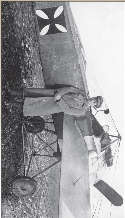
Ernst Preberr von Althaus poses in front of his Fokker E II. Note the wind blown black paint runs from the freshly(?) painted fuselage eisernkreuz, fuel filler cap behind the cockpit, head rest and Garuda propeller. The lag for attaching the wings to the side of the fuselage is barely visible on the far left of the photo. Ernsts appears to have found one of the few dry patches in France to park his Eindecker on.
